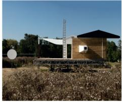
assembled by Vantage Event and Media Structures. The radio equipment and mast were installed once the build was complete. The mast was attached to a scaffold ladder tower at the centre of the station.
